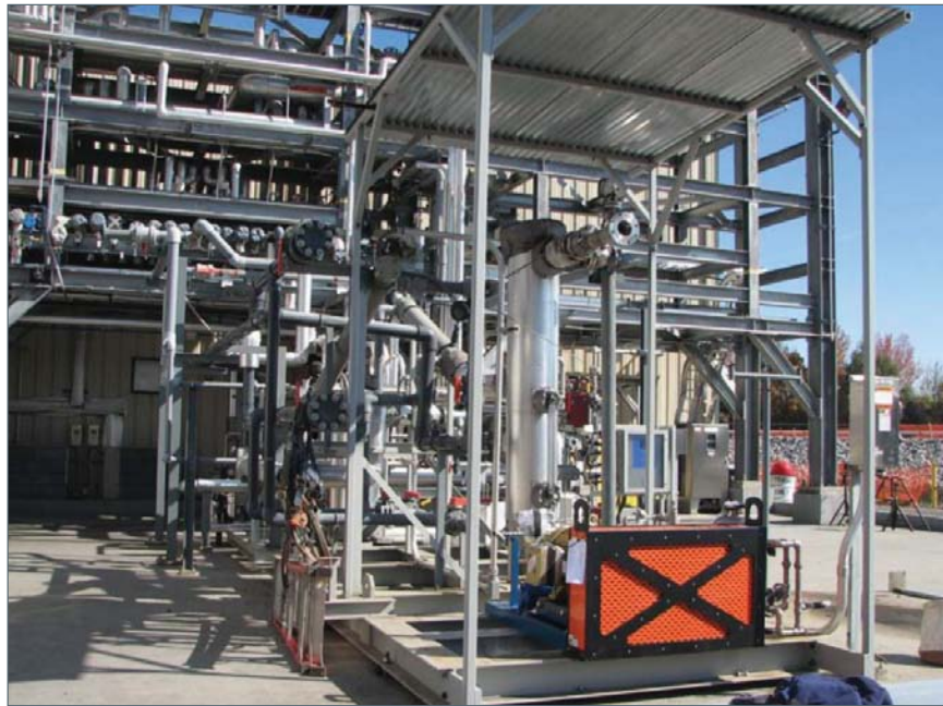
Figure 4: Membrane Skid Used for 1-tpd Bench-Scale Slipstream Testing at NCCC
