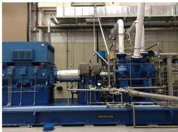
Figure 4. Installed Dresser-Rand Datum Compressor Package
