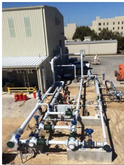
Figure 5. Pipe Loop Assembly Aerial View
